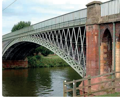
Mythe Bridge, İngiltere 1826, L= 52 m (dökme demir).
