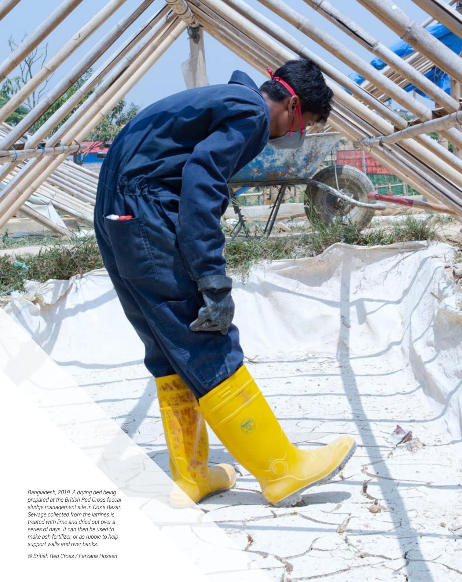
Bangladesh, 2019. A drying bed being prepared at the British Red Cross faecal sludge management site in Cox's Bazar. Sewage collected from the latrines is treated with lime and dried out over a series of days. It can then be used to make ash fertilizer, or as rubble to help support walls and river banks.
